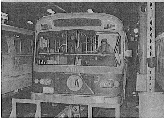
A mechanic checks the air pressure on 4064 in January 1982. Note service pit and support columns to left of the bus. Fifth Avenue's 4000s were well maintained.
