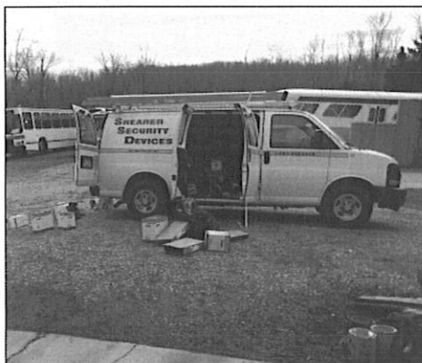
Shearer Security truck installing the alarm system at the annex.
